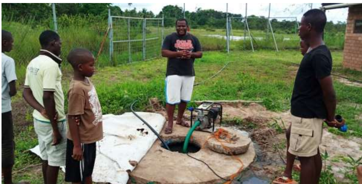
Fixing the water pump
